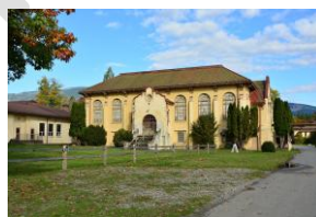
Former Chapel and auditorium of Northern State Hospital, now a conference center. Photo by Joe Mabel.
