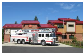
Modern day fire truck in front of fire station. Photo credit Chief Frank Wagner.
