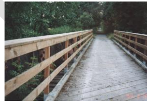
Cascade Trail east of Sedro-Woolley. Photo by Robert Ashworth.
