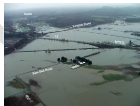
2009 flooding in Skagit County. Photo by WSDOT.
