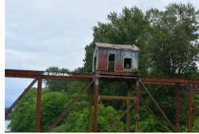
1913 bridge over the Skagit River near Sedro-Woolley. Photo credit Joe Mabel.
