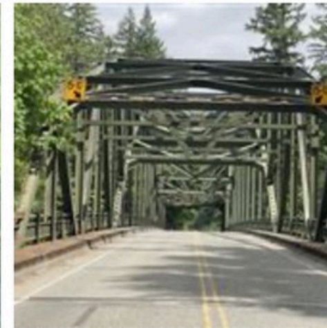
Concrete Sauk Valley Bridge
