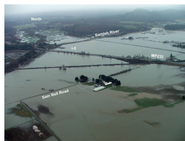
2009 flooding in Skagit County. Photo by WSDOT.
