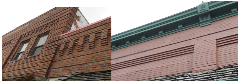
Examples of remnant dentil detailing (left) and crown molding (right) in Sedro-Woolley’s CBD.
