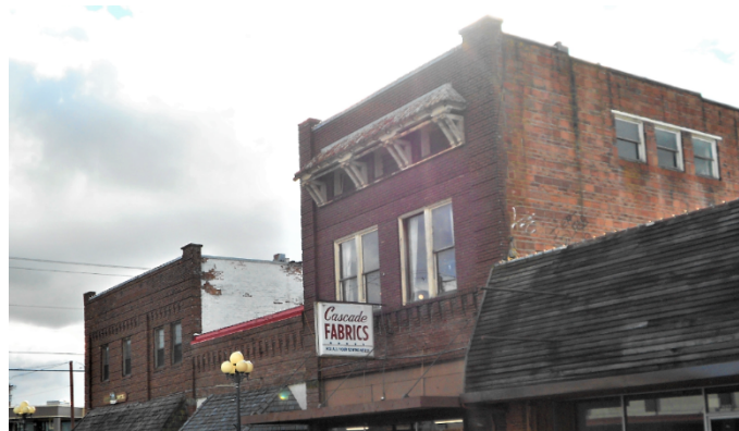
Examples of historic Art Nouveau style architecture in downtown Sedro-Woolley displaying tall, decorative fronts.
