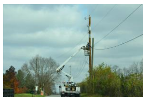
Electricians working on fiberoptic cable. Photo by Roger Starnes Sr.
