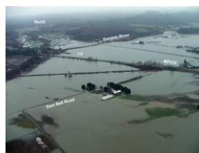
2009 flooding in Skagit County. Photo by WSDOT.
